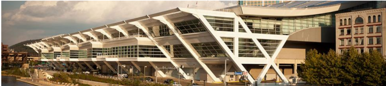
View of the convention center from the river
