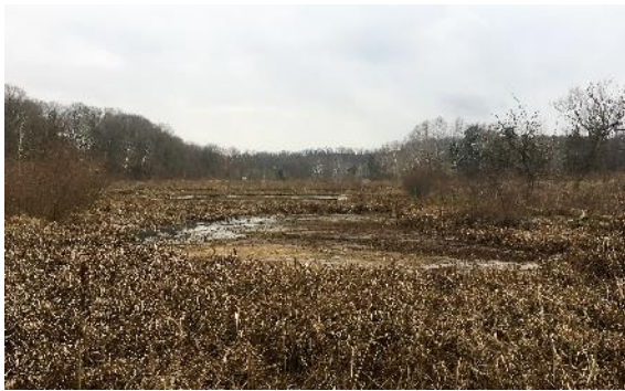
Passive wetland treatment system for drainage from an abandoned coal mine
