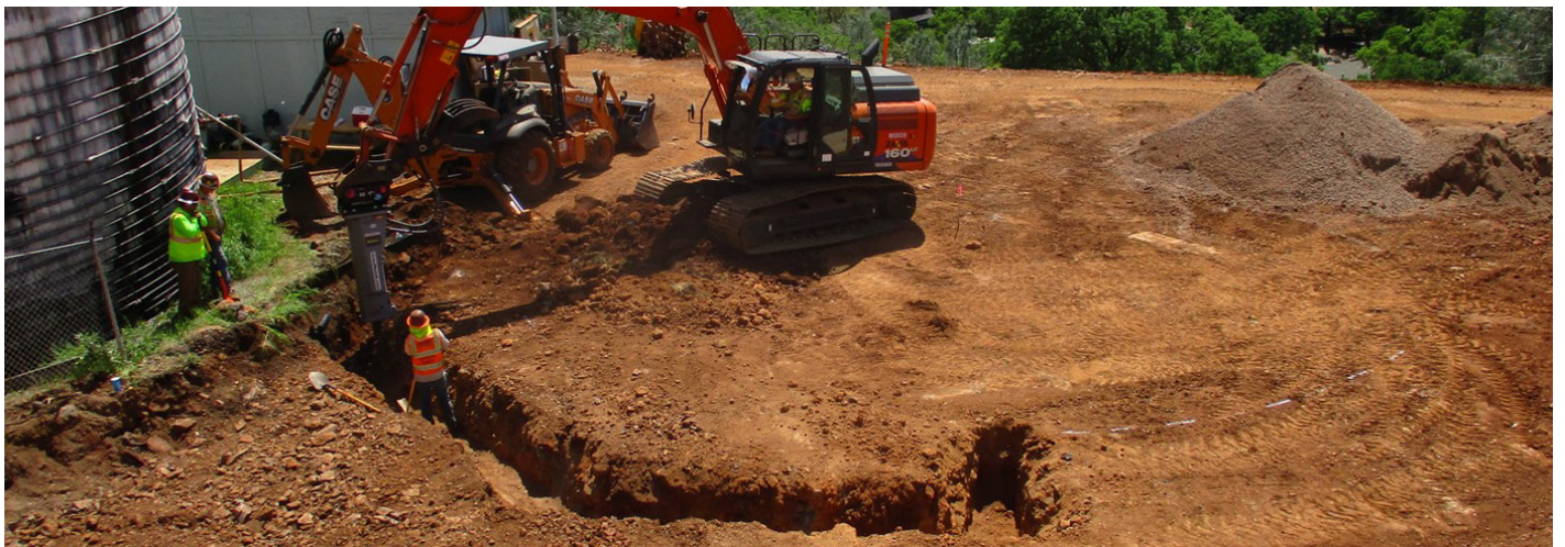
Hidden Valley Lake CSD Water Tank Replacement, excavation of the foundation.
