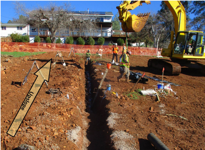
Back feed trench
