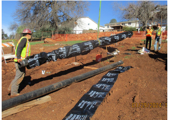
Back feed pipe installation.
